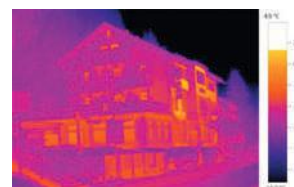
Thermal image with ScaleAssist
